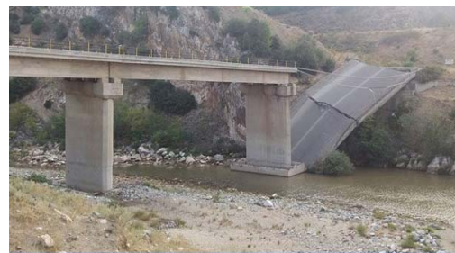
Figure 1: Bridge failure due to flood, causing deck unseating at Trikala, Kalamapaka. Bridge failure due to foundation failure (rotation) at Iasmos, Rodopi.
