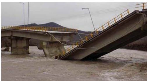
Figure 1: Bridge failure due to flood, causing deck unseating at Trikala, Kalamapaka. Bridge failure due to foundation failure (rotation) at Iasmos, Rodopi.
