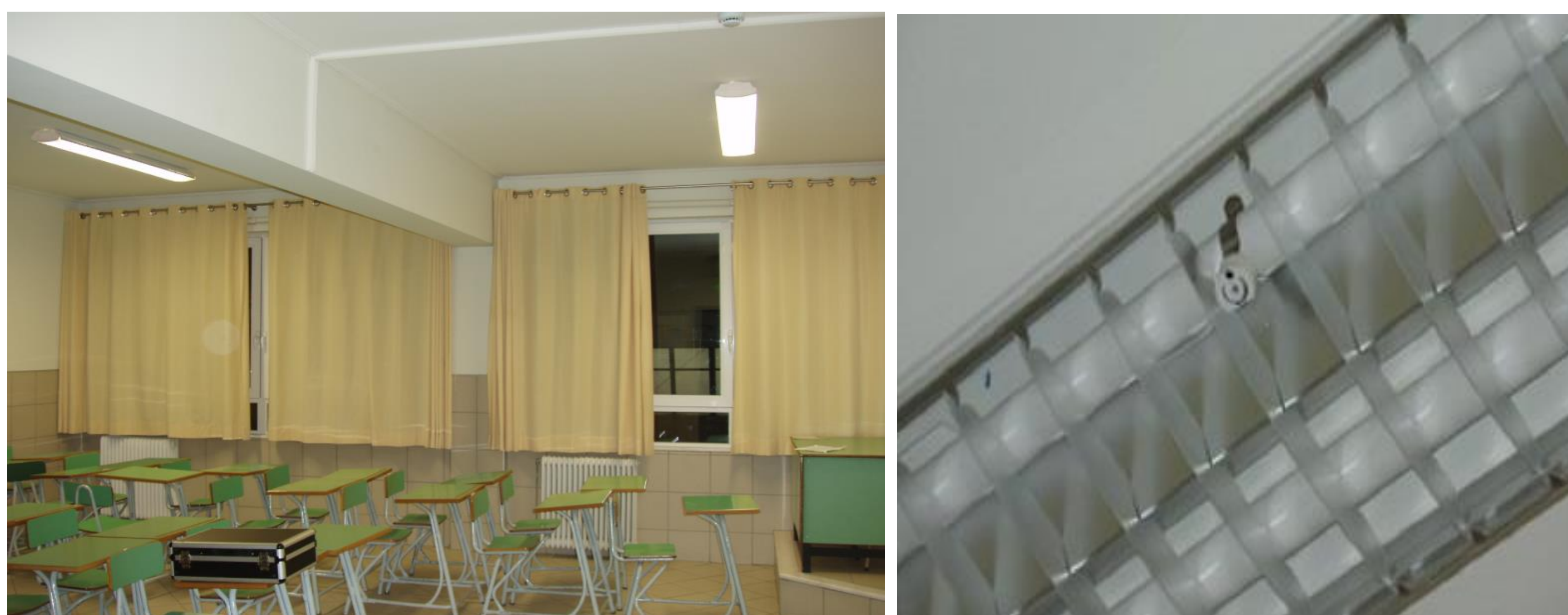
Figure 2. Left: Classroom A with the installed photosensors during the nighttime commissioning [4, 5]. Right: The installed standalone photosensor using integral-reset algorithm
