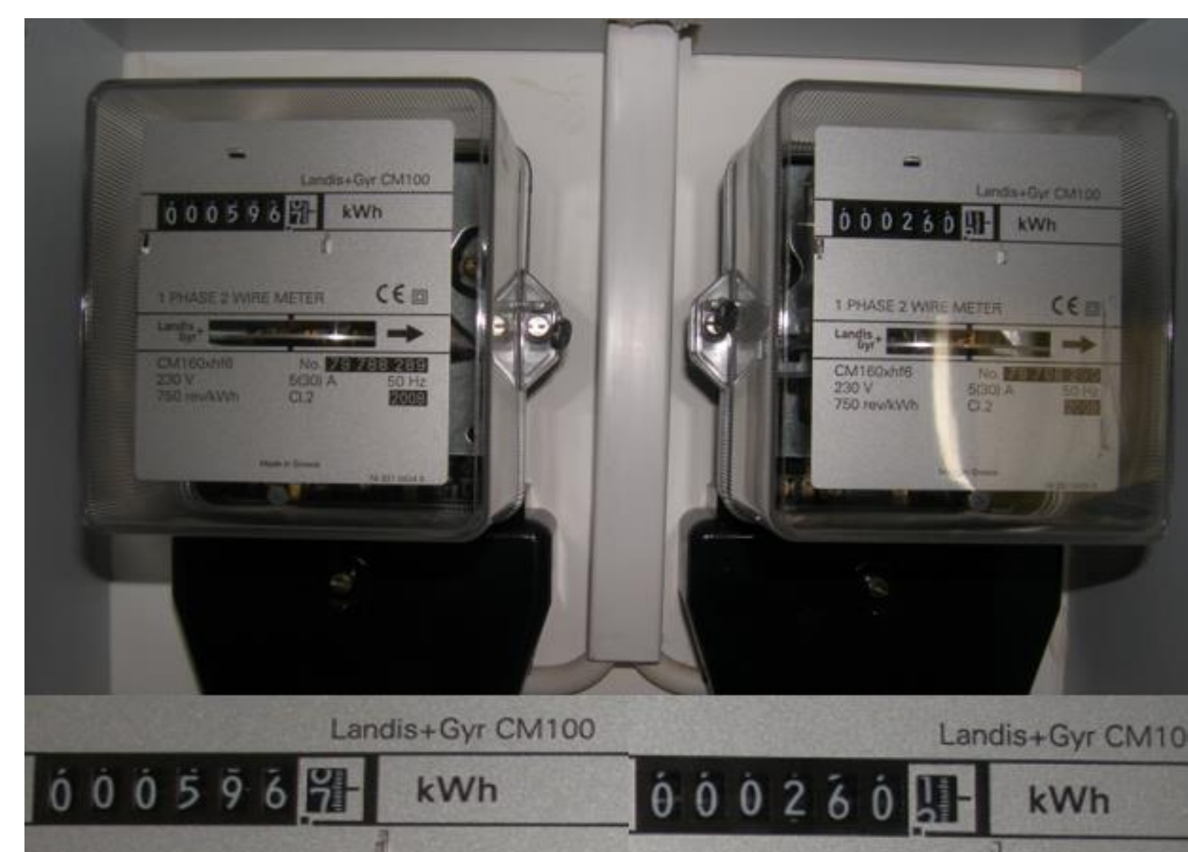
Figure 3. The metering equipment and the corresponding results from the first year of implementation. Left: Energy consumption of classroom B (Electricity kWh). Right: Energy consumption of classroom A using photosensors for daylight harvesting (Electricity kWh).
